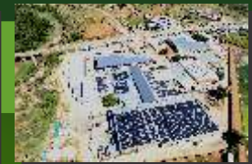
Steilloop Shopping Centre Phase 2
